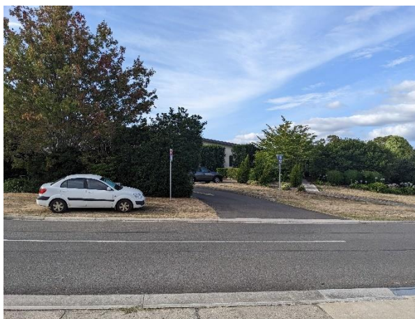
Figure 9: Trees blocking sight distance at Goodstart Early Learning
